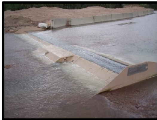
Figure 4-5: Bedload Collector
