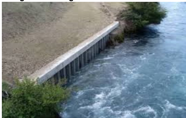
Using Sheet Piling
