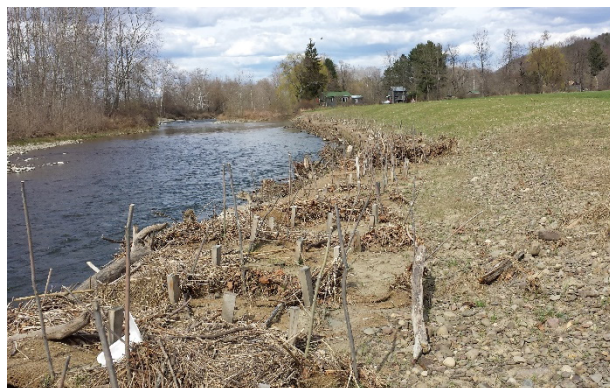
Bank Protection using Logs and Vegetation
